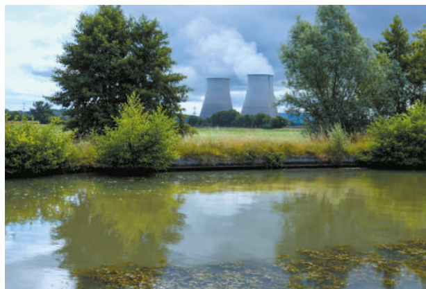
© Gilles P. - Centrale Electrique, Dampierre-en-Burly (45).
